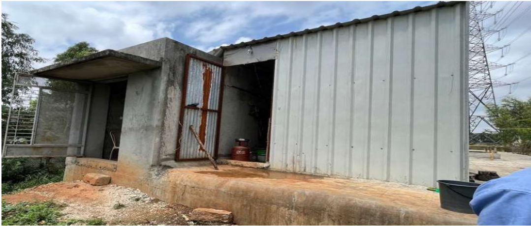
Sewage Treatment Plant 300 KLD
