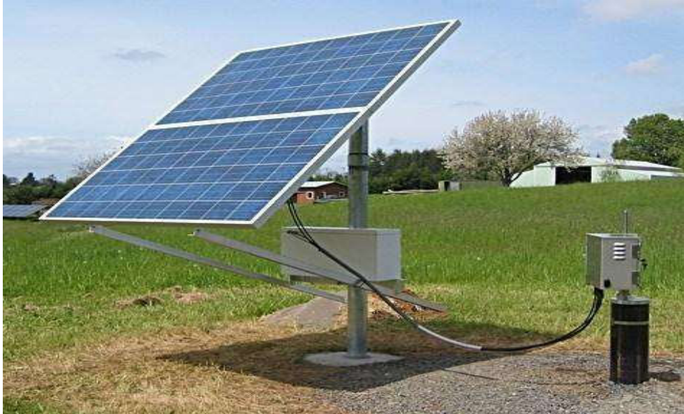
Figure 22: Solar water pump
