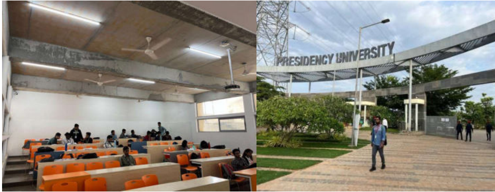
Energy efficient street lights (Presidency University, Bangalore, India)
