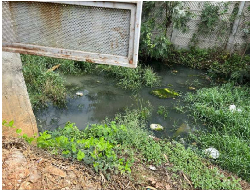
Sewage Treatment Plant (Presidency University, Bangalore, India)
