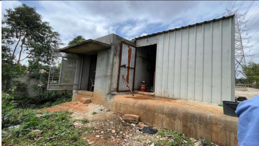
Sewage Treatment Plant 300 KLD (Presidency University, Bangalore, India)
