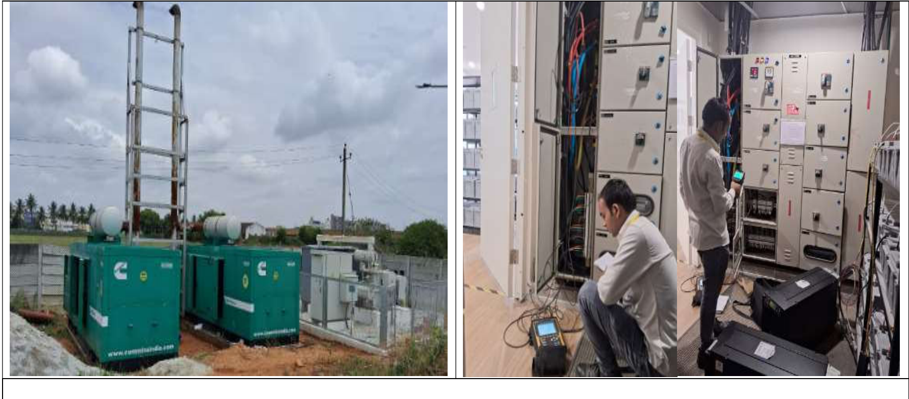
Figure 6: Site visit and measurement in DG loading analysis
